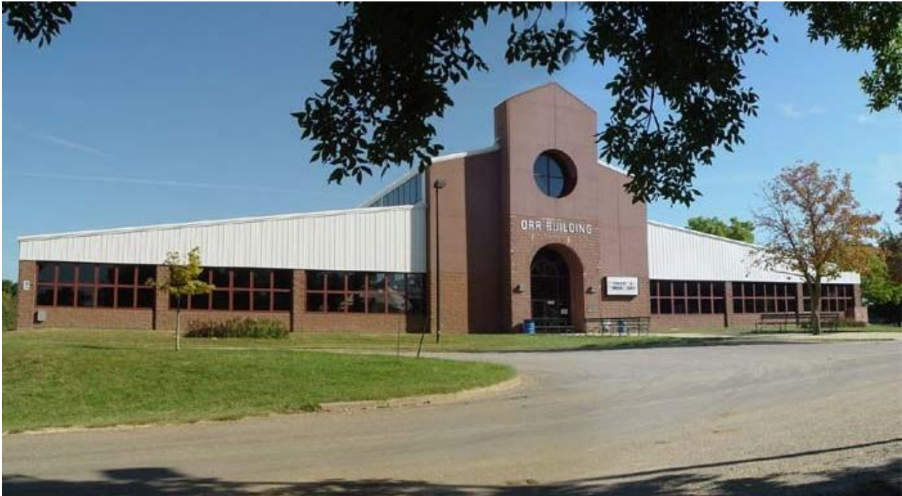
Front view of the Orr Building
